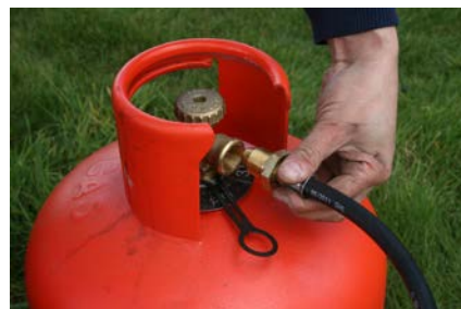
7. Offer up the tail to the second gas bottle and hand tighten in the same way. Make sure the tail is not stretched.
